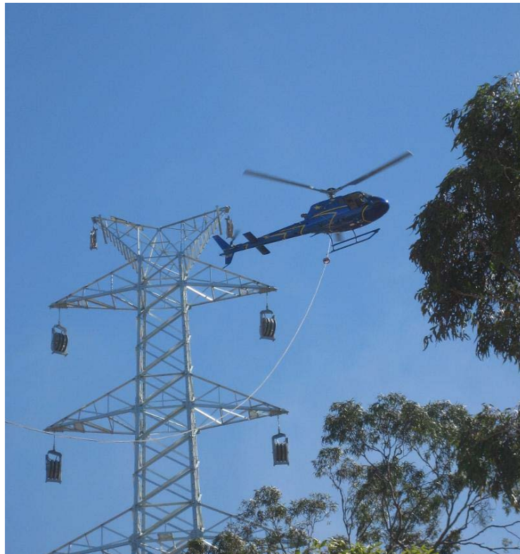
Plate 3-2 Stringing sheaves and helicopter stringing
