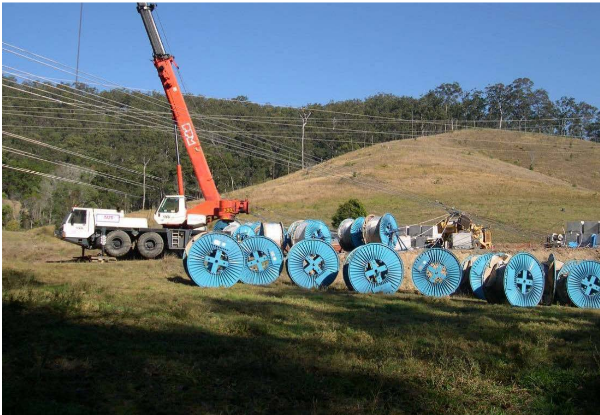
Plate 3-1 Transmission conductor drums and mobile crane utilised in structure erection
