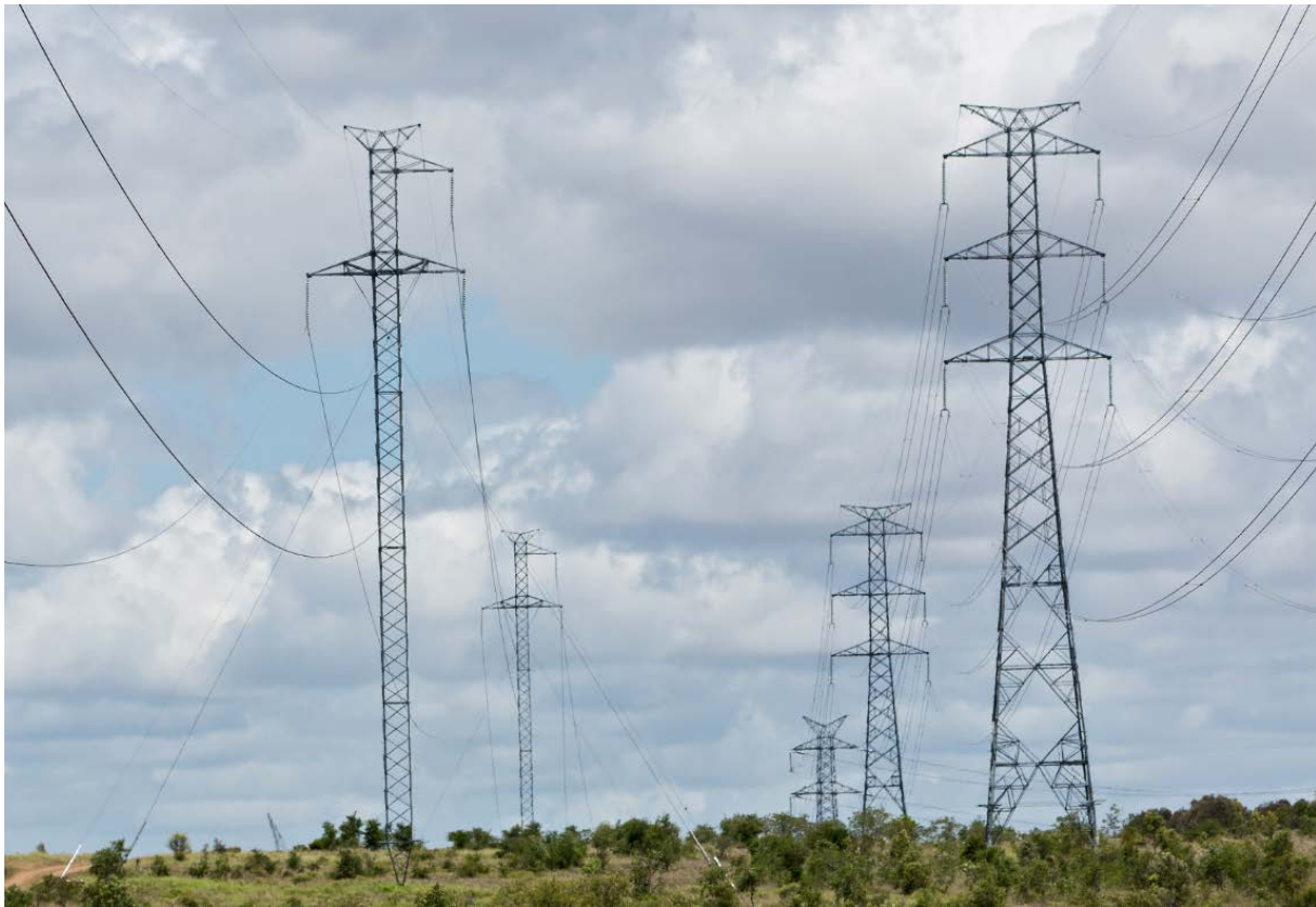
Figure 3-3 Structure types – single circuit guyed structure (left); self-supporting double circuit structure (right)
