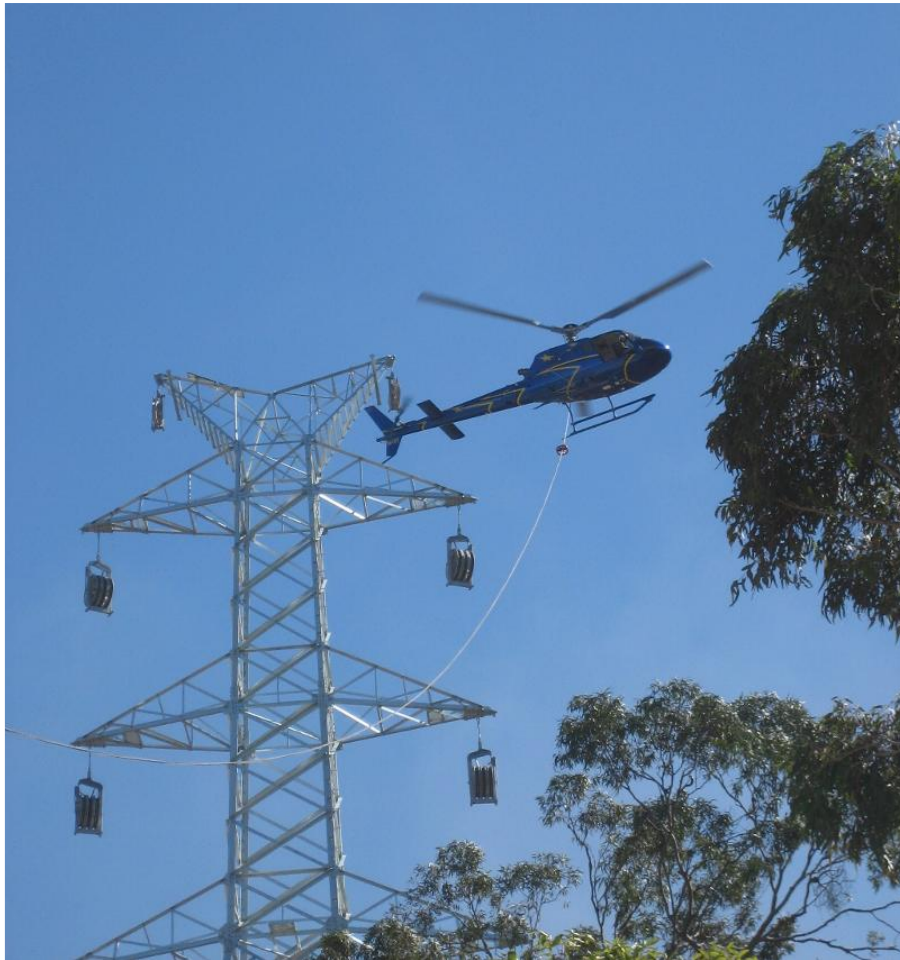
Plate 3-2 Stringing sheaves and helicopter stringing
