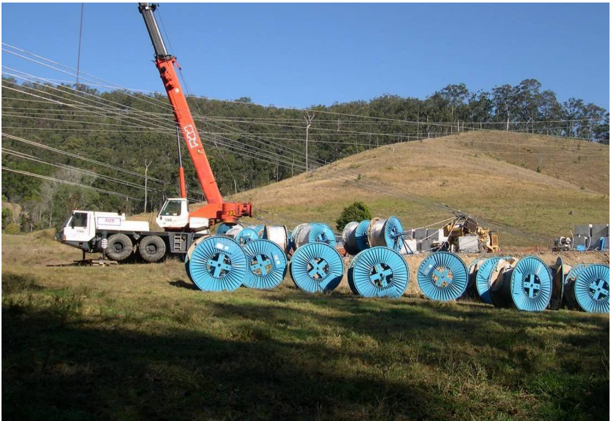
Plate 1-1 Transmission conductor drums and mobile crane utilised in structure erection
