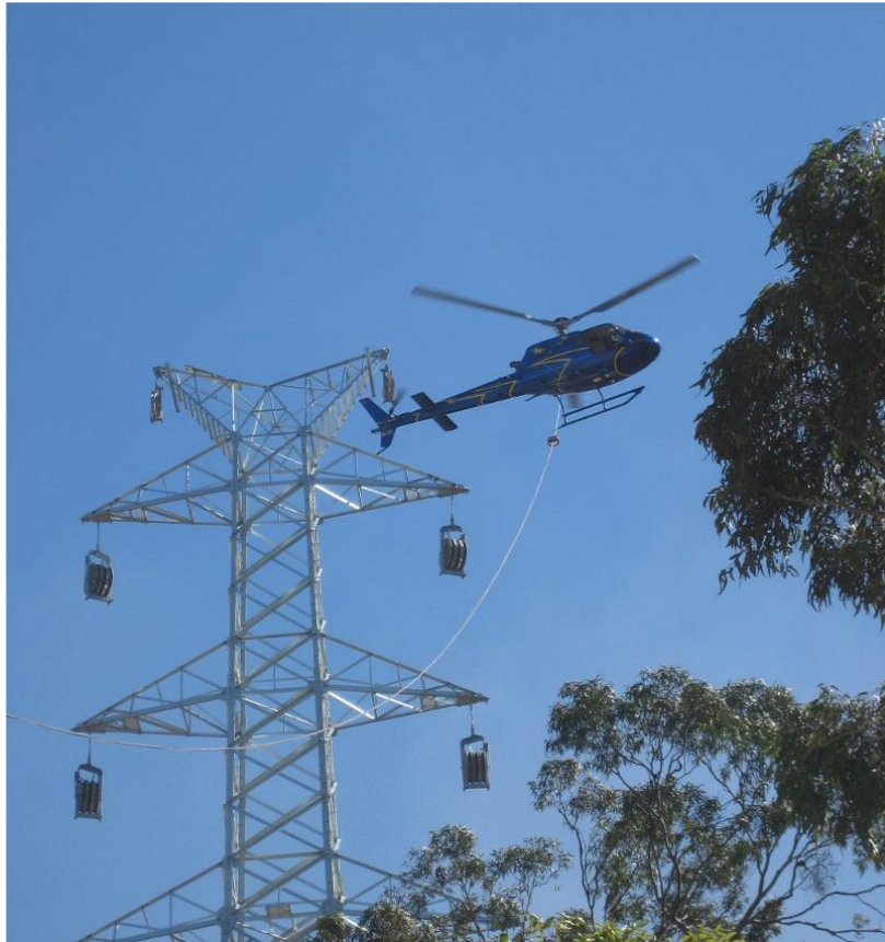
Plate 1-2 Stringing sheaves and helicopter stringing
