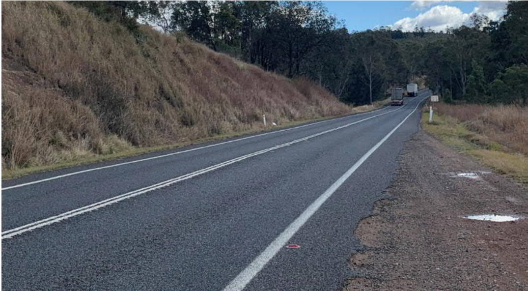
Photo 4.3 D'Aguilar Highway between Yarraman and Tarong Power Station Road facing north Tarong Power Station Road
