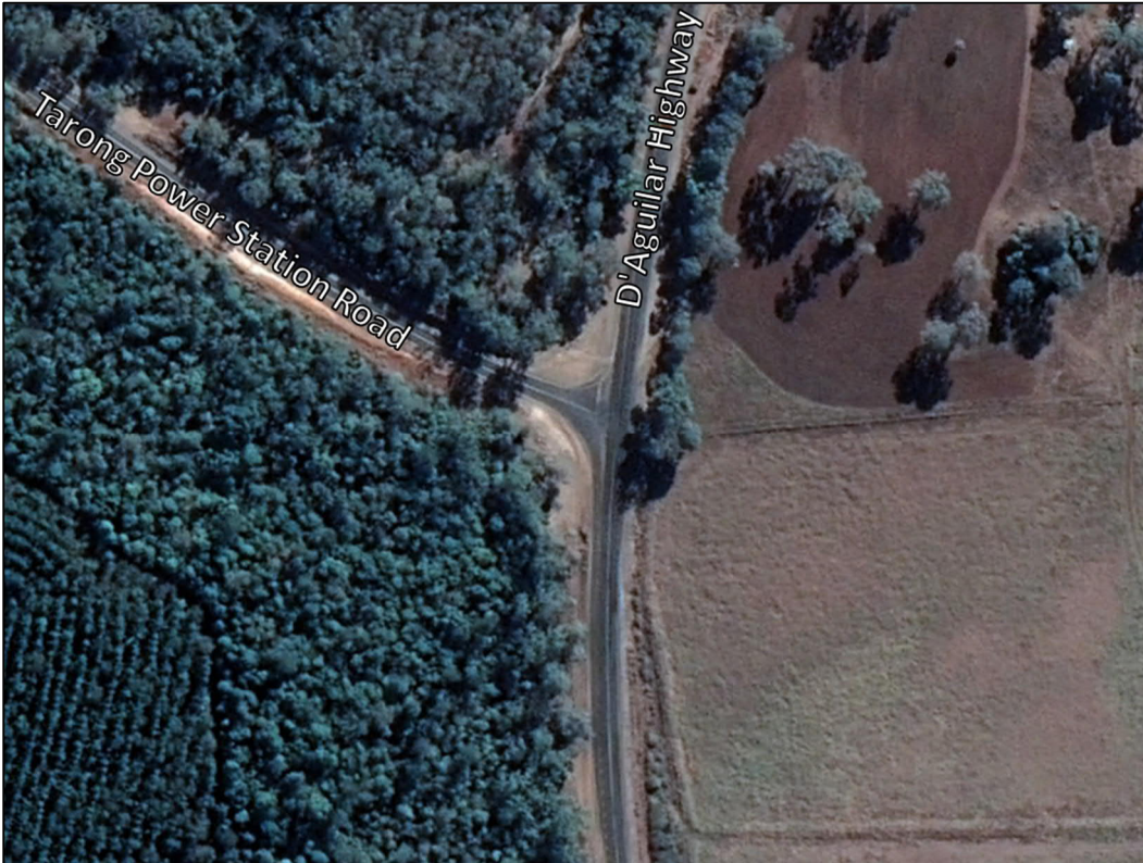
Figure 3.3 D'Aguilar Highway / Tarong Power Station Road intersection (source: Google Earth)
