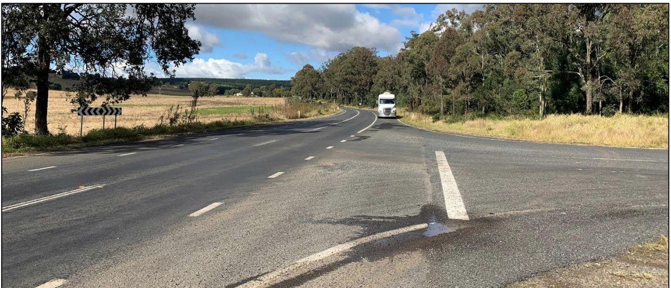
Figure 3.4 D'Aguilar Highway / Tarong Power Station Road intersection (facing south)
