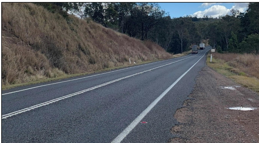
Figure 3.1 D’Aguilar Highway between Yarraman and Tarong Power Station Road facing north
