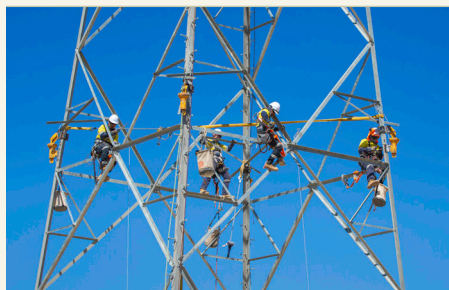
Transmission tower assembly in progress.
