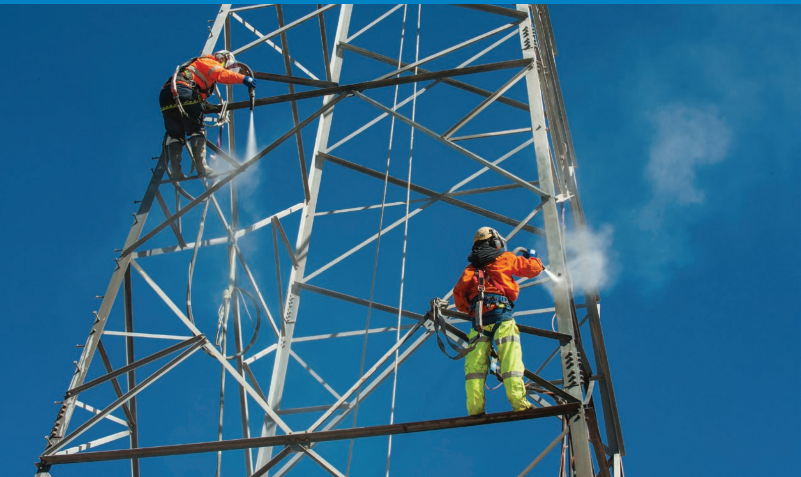
Abrasive blasting taking place on the Runcorn to Belmont transmission line as part of refit activities to safeguard network reliability.
