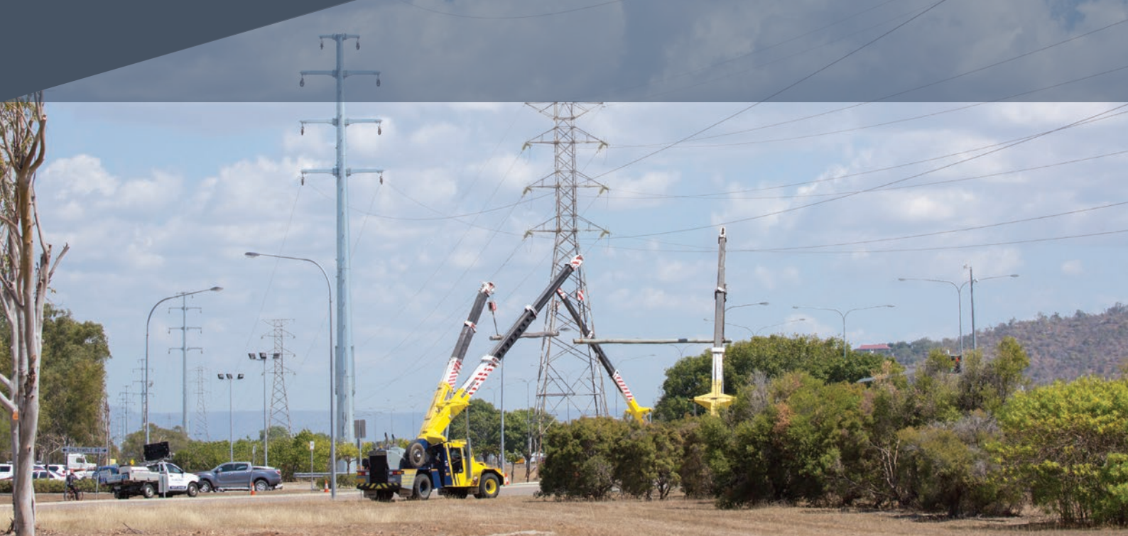
Replacing the ageing Garbutt to Alan Sherriff transmission line to maintain a safe and reliable electricity supply to the Townsville region.
