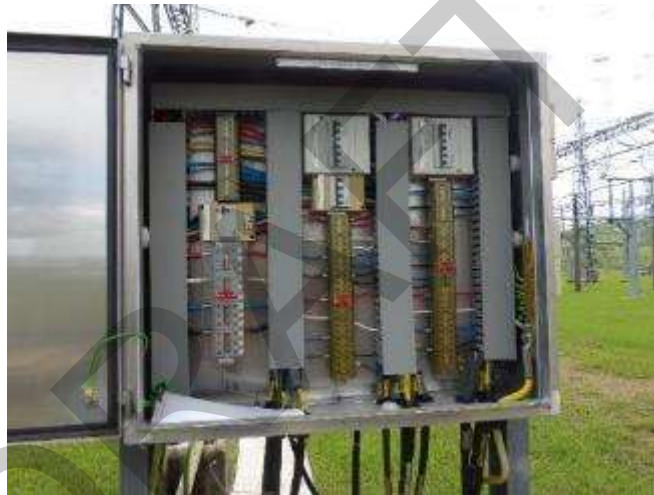
(b) =D07-A92 Bay DC Marshalling Kiosk
