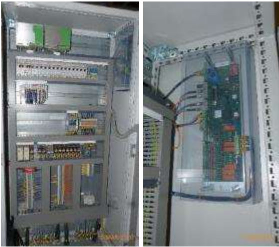
Figure 11 – SVC Cooling Control System Panel
