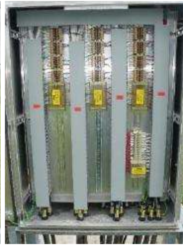
(a) =D03-A10 Bay Marshalling Kiosk
