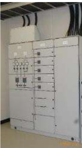
SVC 400V AC Auxiliary / Changeover Panel
