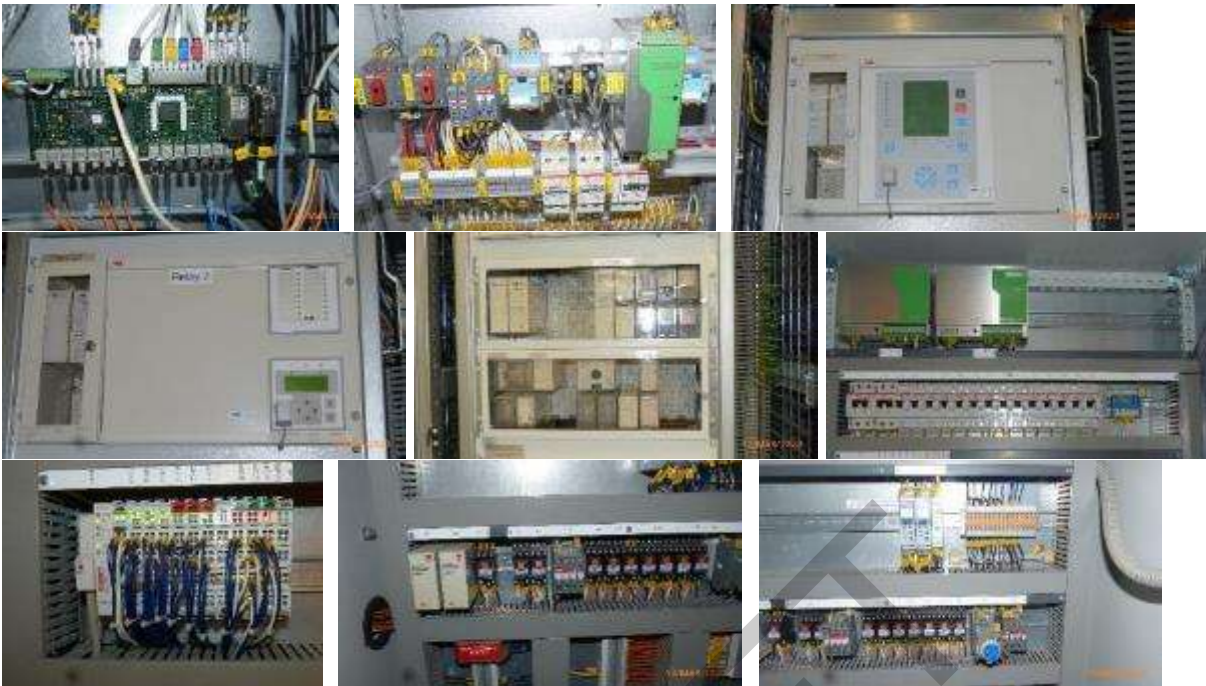
Figure 13 – Woollooga SVC Typical SVC Indoor Secondary System Equipment (2008)
