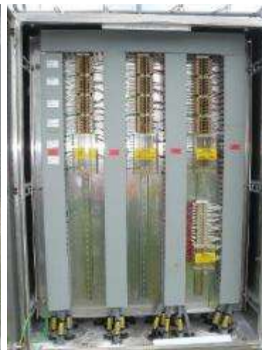
(c) =D18-A10 Bay Marshalling Kiosk
