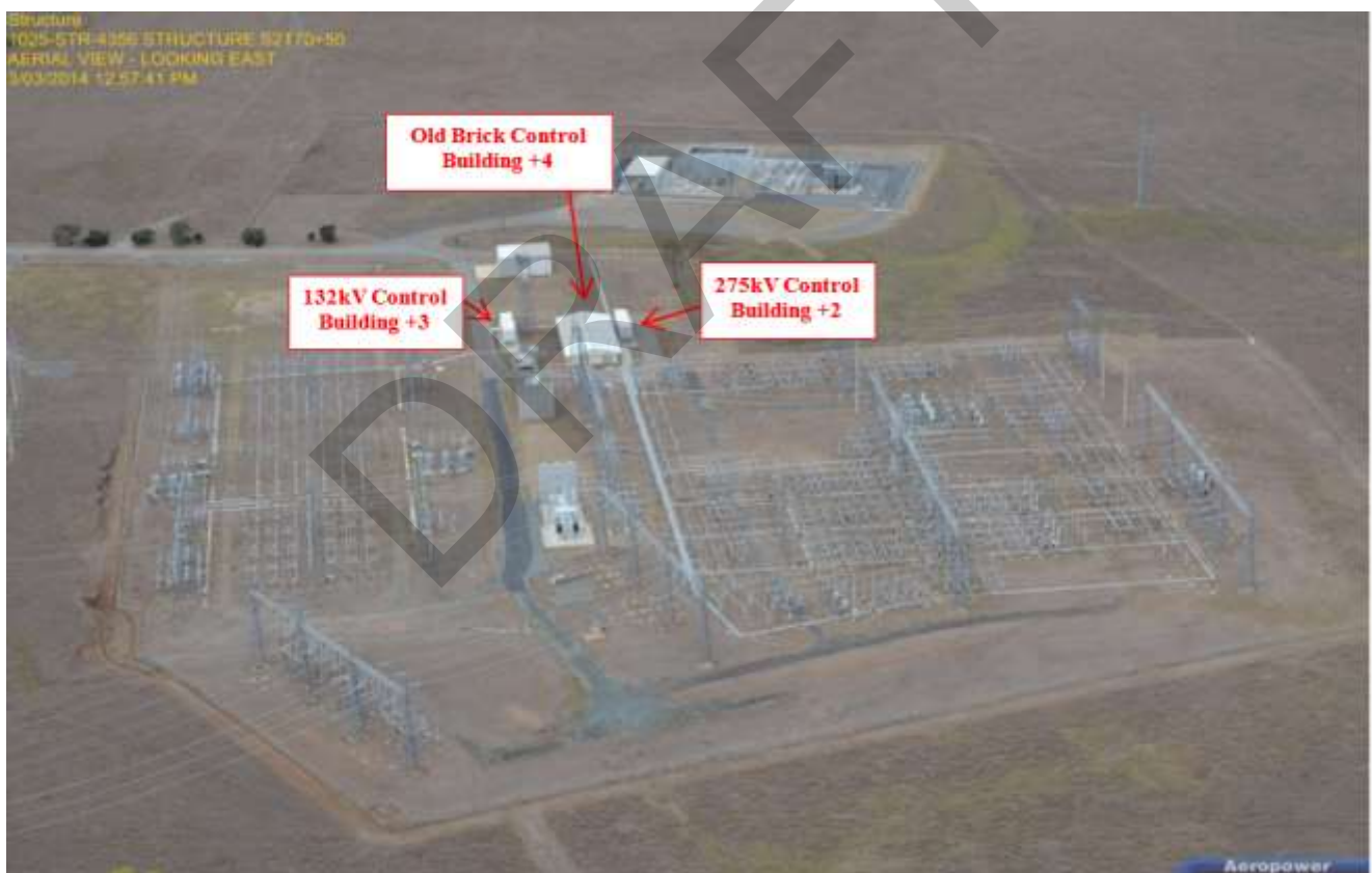
132kV/275kV Woolooga Substation control room arrangement
