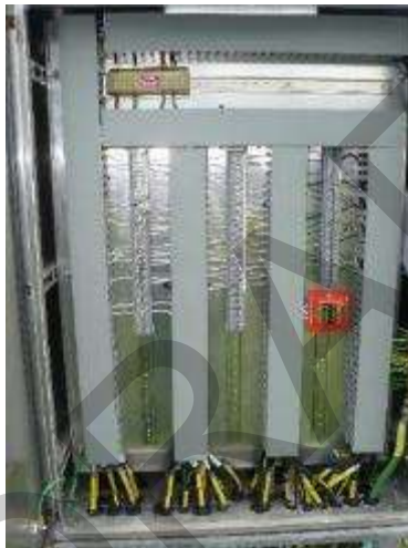
(b) =D11-A10 Bay Marshalling Kiosk
