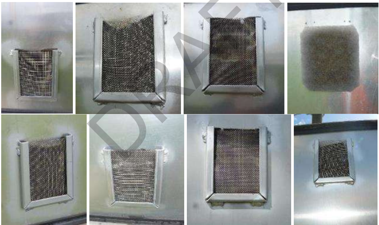
Figure 6 – Physical appearance of typical outdoor marshalling kiosks air filters at Woollooga substation
