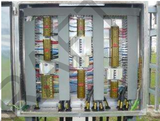
(e) =C01-A91 Bay AC Marshalling Kiosk
