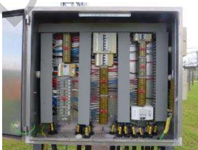
(c) =D15-A91 Bay AC Marshalling Kiosk
