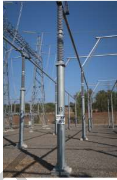
Figure 18: 275kV Tubular Bus Support Structure
