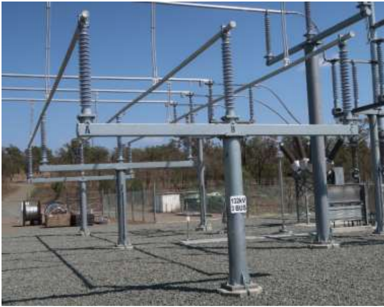
Figure 17: 132kV Bus Support Structure
