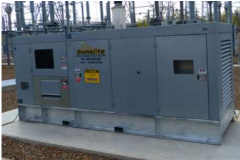
Figure 25: Diesel generator
