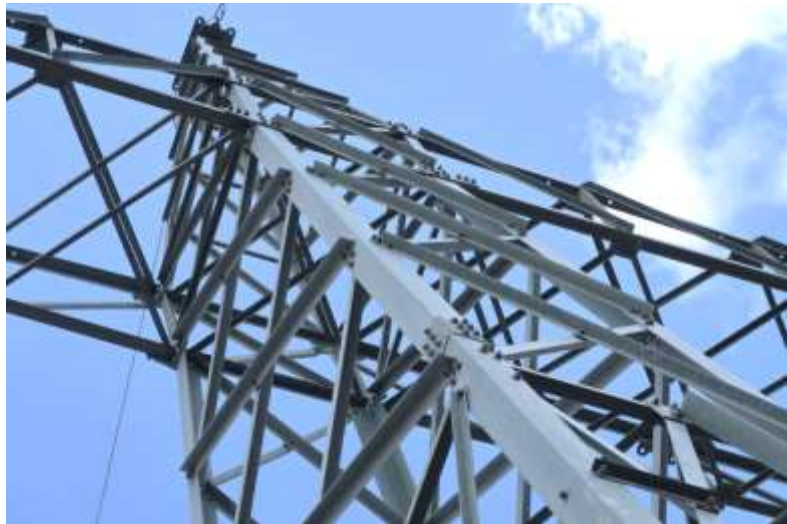
Figure 22: 275kV Structure Main Leg
