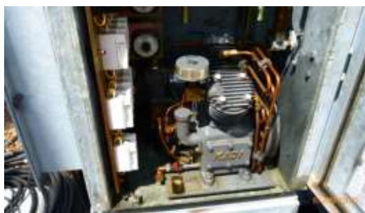
Figure 14: CB Mech box oil leak
