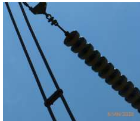
Figure 20: strung bus conductors
