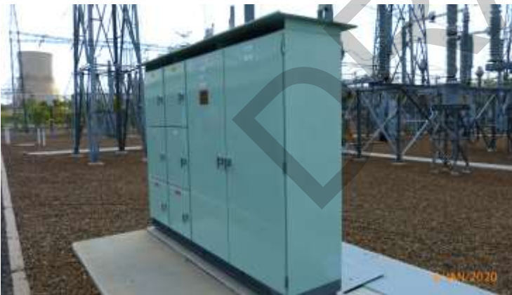
Figure 26: AC changeover board
