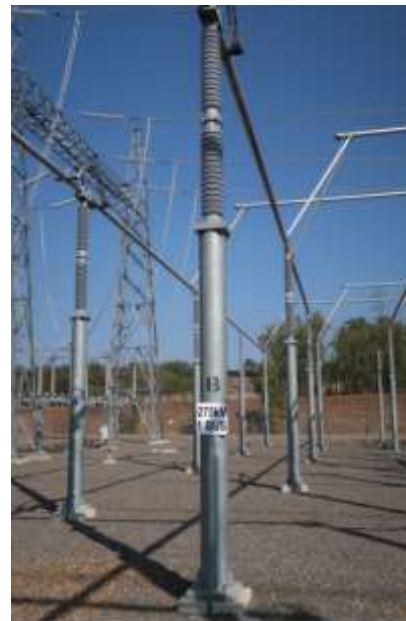
Figure 16: 275kV Tubular Bus Support Structure
