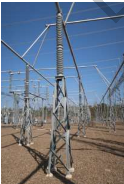
Figure 15: 275kV Lattice Bus Support Structure
