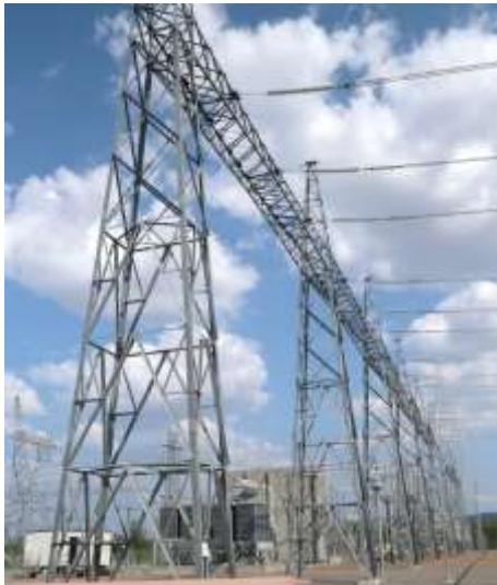
Figure 21: 275kV Strain Structure
