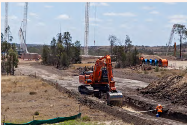
5. Excavating drains if required.
