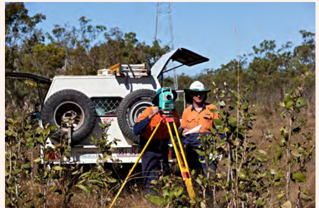
2. Marking the exact position for each transmission structure (i.e. steel lattice tower or pole).
