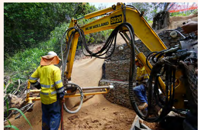
6. Stabilising any new embankments (batters).
