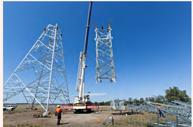
2. Steel lattice towers may be erected using cranes and elevated work platforms.
