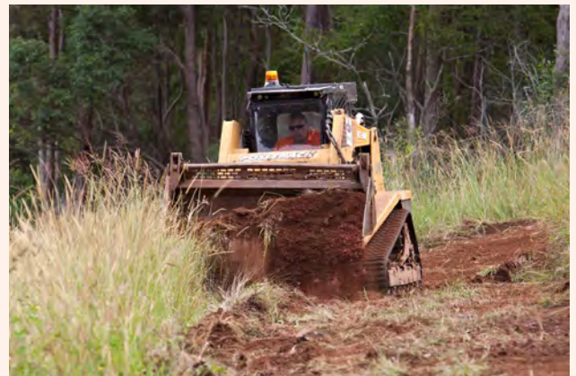
4. Preparing tower sites and associated access tracks.
