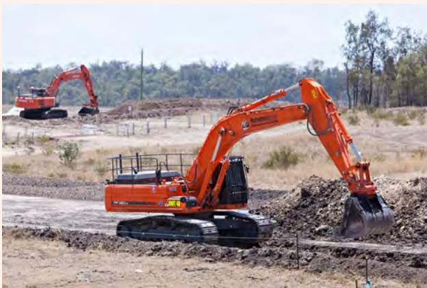
3. Trenches and roadways are excavated.
