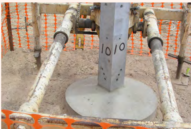
3. The necessary steelwork is inserted and the foundation is completed.
