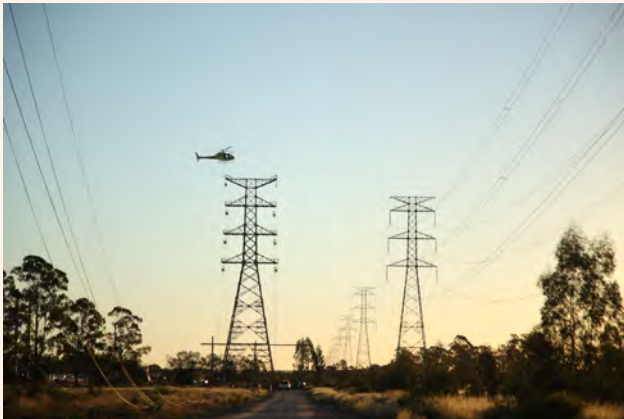
Helicopter Aerially strings transmission lines.
