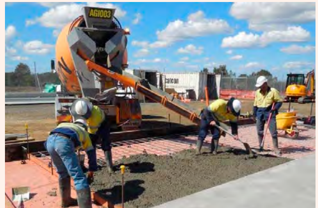
2. Concrete is poured and left to cure, which completes the foundation.
