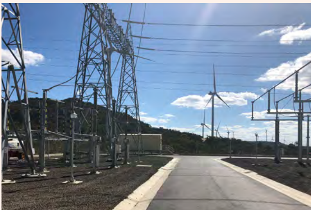
3. Internal roads are sealed and gravel is laid on the remainder of the substation site.
