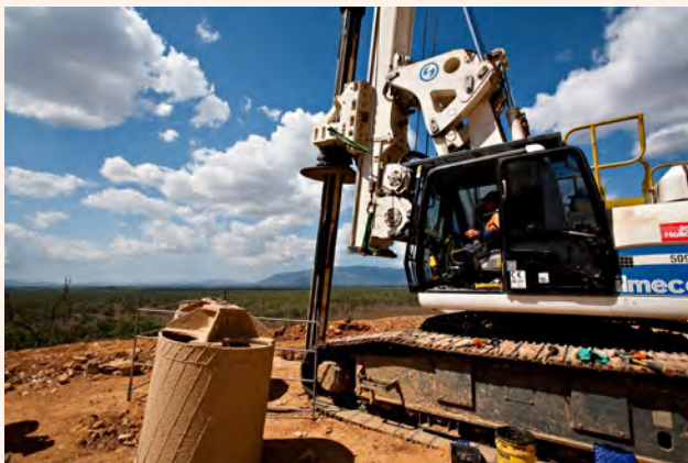
1. A large boring machine is used to excavate foundations which can be up to 10m deep and 1.4m in diameter.
