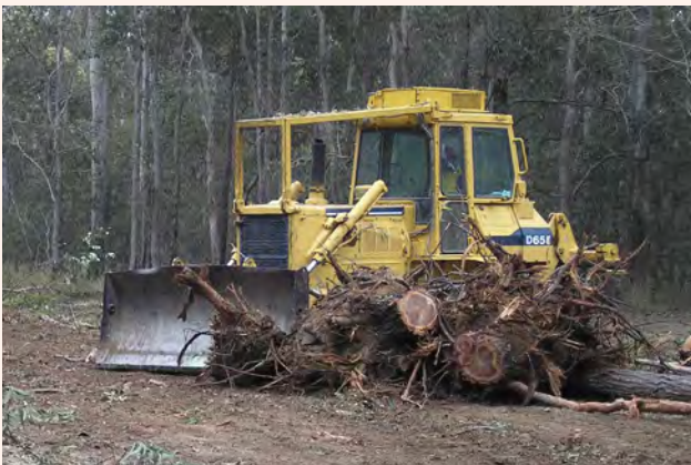
3. Clearing vegetation and preparing tower pads, lay-down areas and general access tracks.
