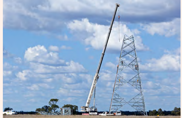
Crane Assembles transmission structures and equipment.
