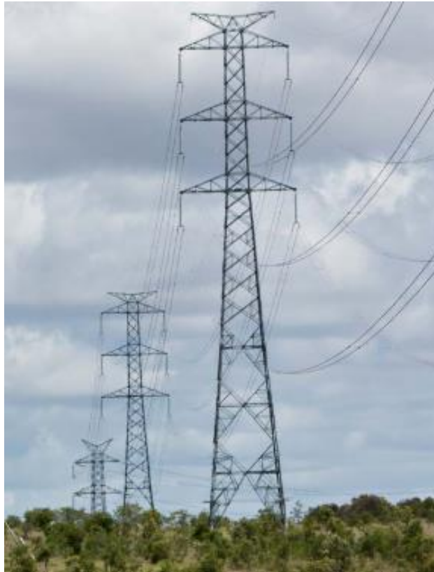
Photo 1 Self-supporting steel lattice tower in double circuit configuration
