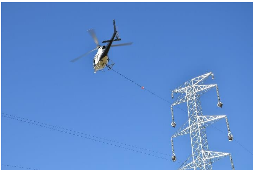
Figure 3.4 Helicopter stringing
