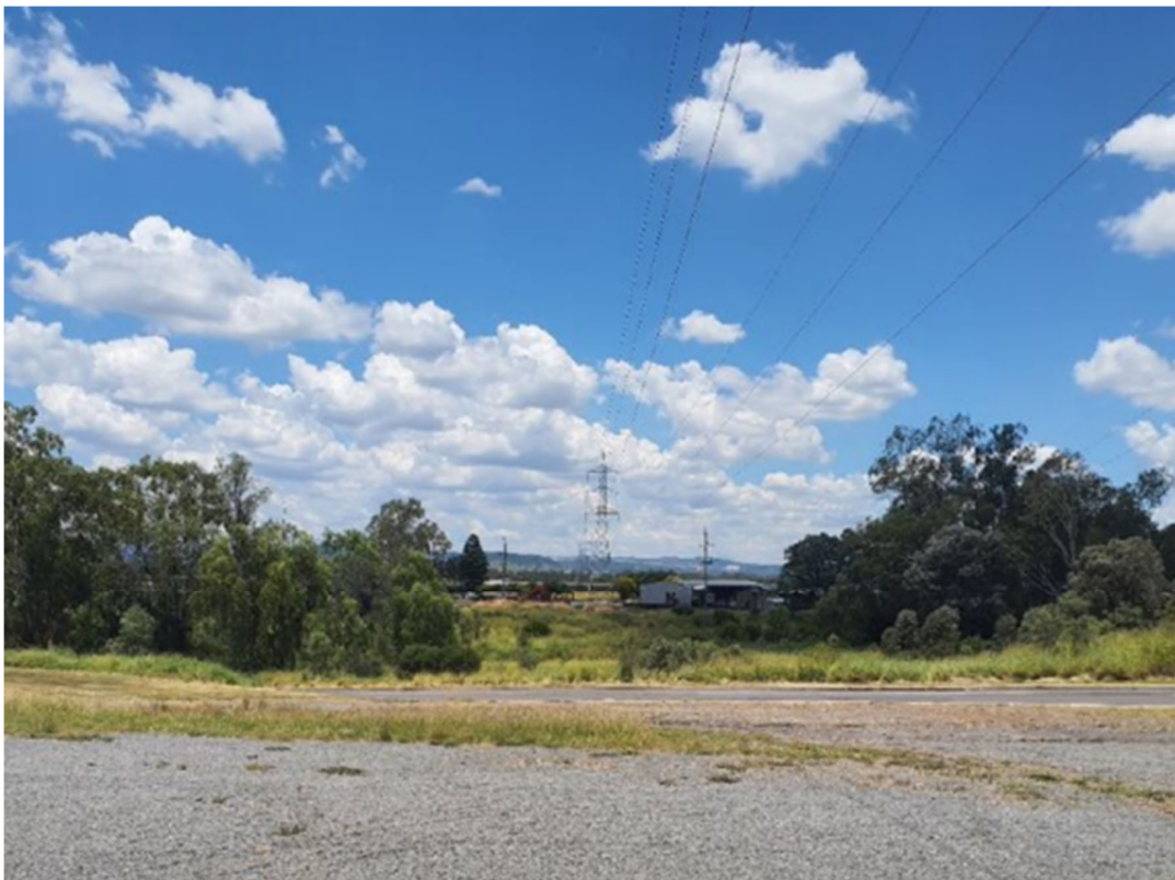
Photo 15 View northeast along State Farm Road with interface between existing 132 kV line and Ergon distribution line
