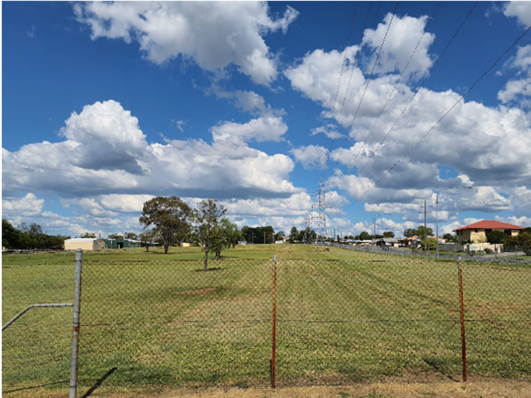
Photo 14 View east along existing 132kV line along Auburn St
