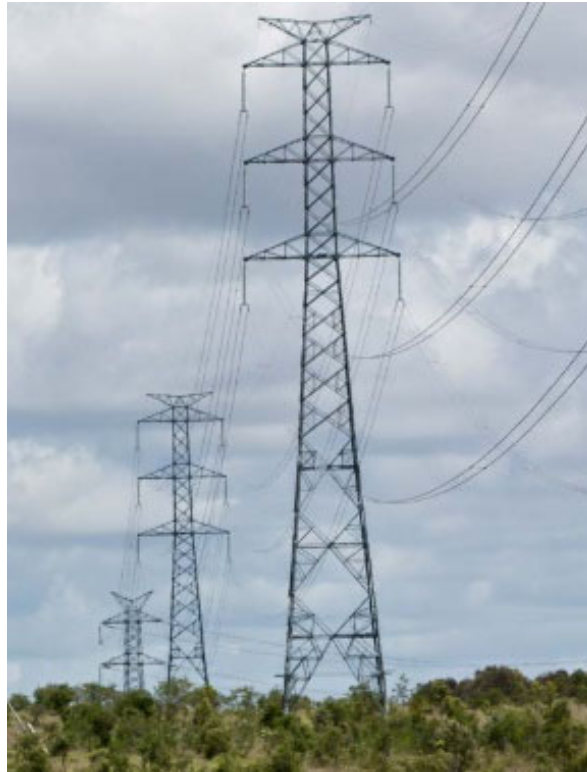
Photo 1 Self-supporting steel lattice tower in double circuit configuration
