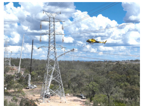
We work with landholders to provide advance notice all works including transmission line stringing by helicopters.
