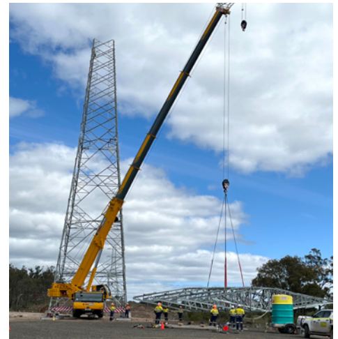
Towers are assembled and installed in sections.
