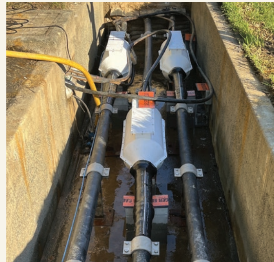
An excavated joint bay
