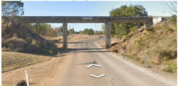
The vertical/horizontal geometry of the Flinders Highway (14B) at an approximate chainage of 0km (around the Rainbow Road / Armstrong Road Flinders Highway intersection) has a rollover risk for over height and over mass vehicles. This should be taken into consideration.
