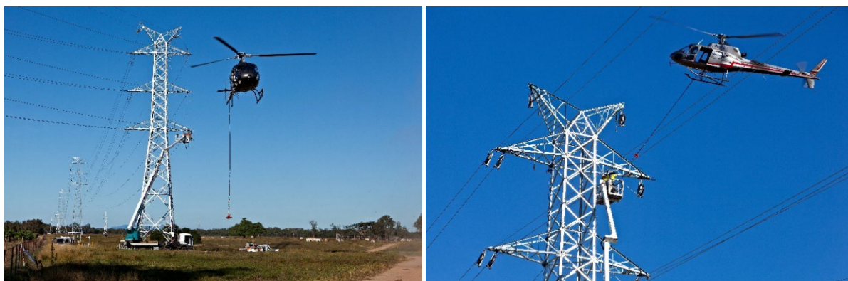
Plate 5 Stringing sheaves and helicopter stringing
