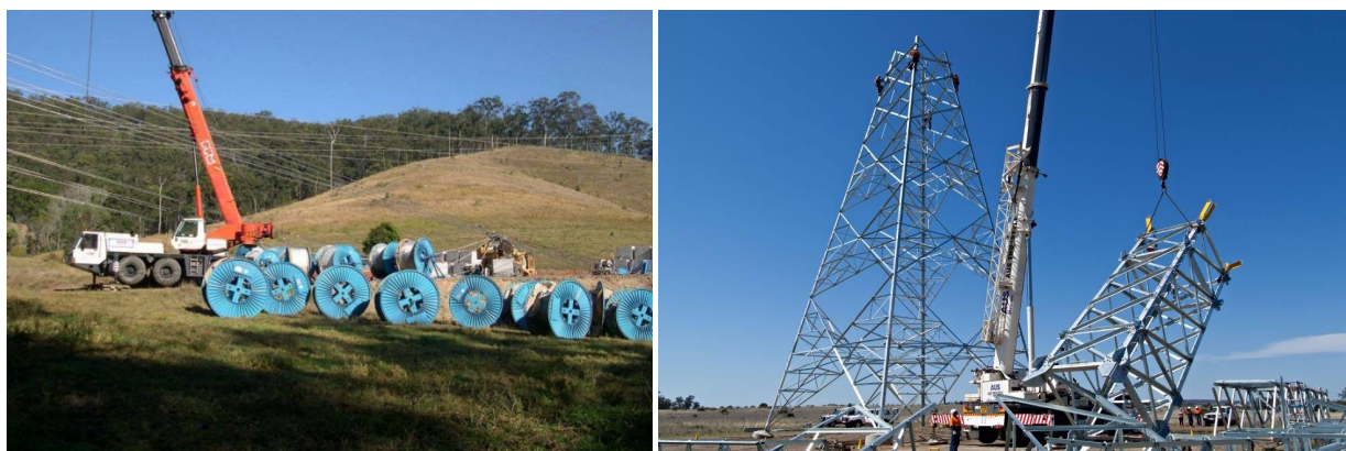
Plate 4 Transmission conductor drums and mobile crane utilised in structure erection
