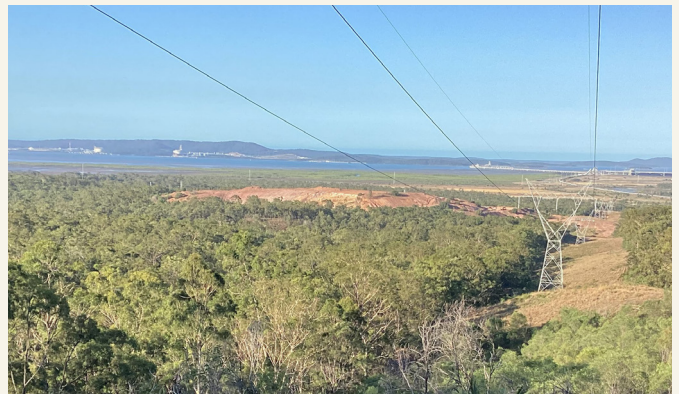
Existing transmission infrastructure near Gladstone. It shows the area under the lines that must be kept free of large-growing trees to manage bushfire risk.
