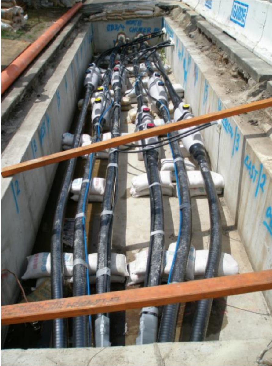
Figure 3-2 Example of a joint bay under construction
