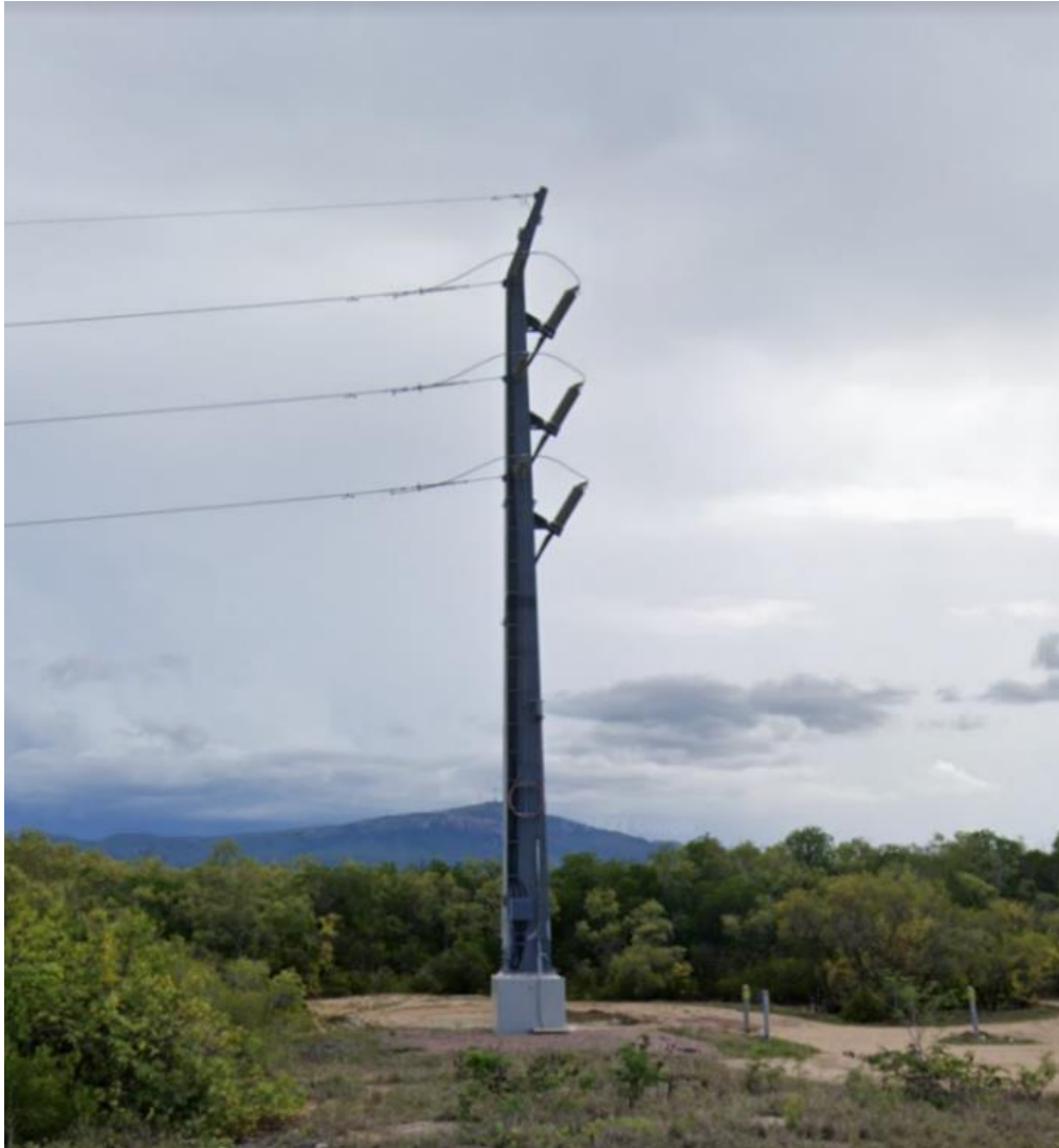
Figure 3-3 Example of an underground to overhead structure
