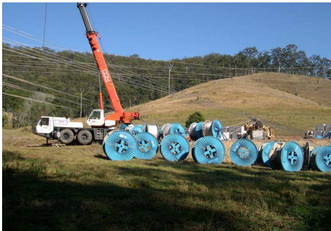
Figure 2.4 Transmission conductor drums and mobile crane utilised in structure erection
