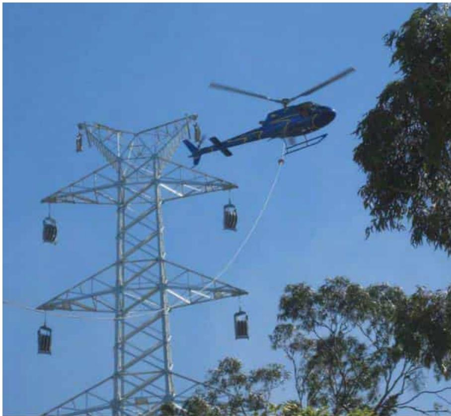
Figure 3.6 Stringing sheaves and helicopter stringing
