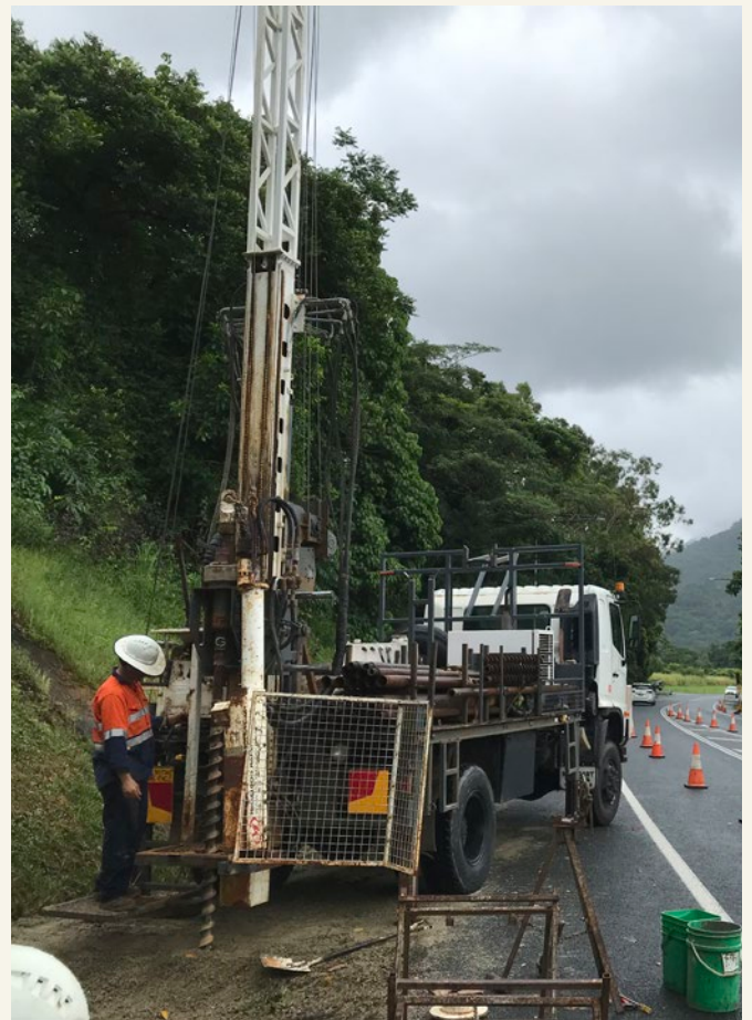
Bore hole testing using a truck mounted drill rig.
