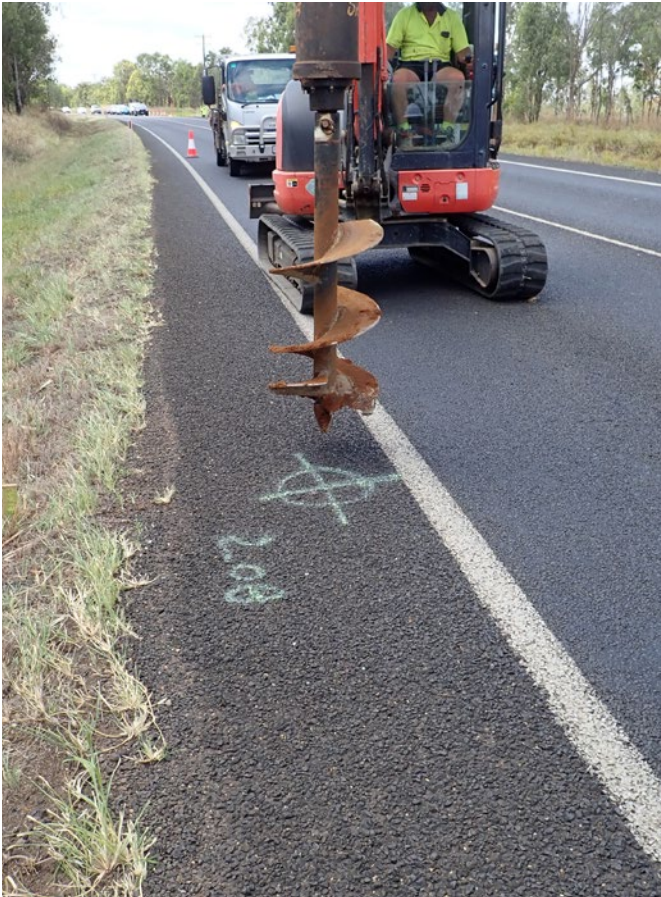
Test pit excavation using a small excavator with an auger attachment.
