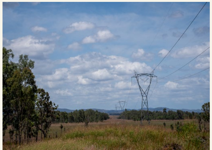
Initial on-site activities will start from July 2026 to prepare the transmission easement for the clearing and access works.
