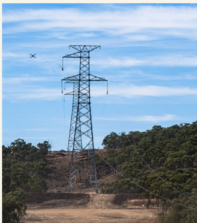
Drone stringing completed for Lotus Creek Wind Farm connection.
