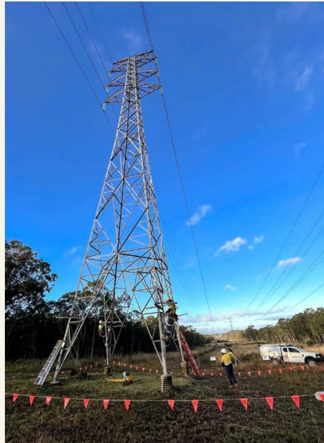
Crews preparing the works area.
