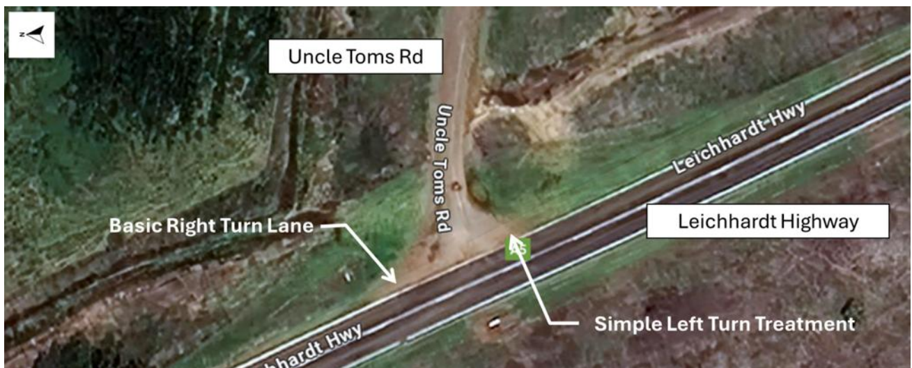
Figure 18.7 Leichhardt Highway/Uncle Toms Road intersection
