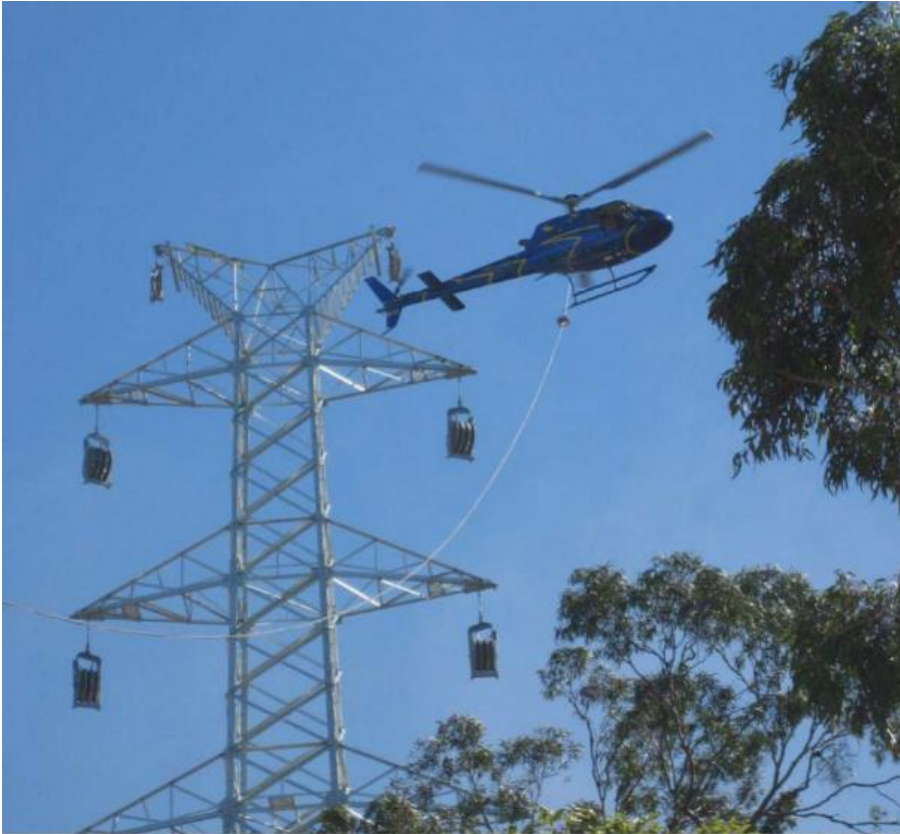
Figure 3.6 Stringing sheaves and helicopter stringing
