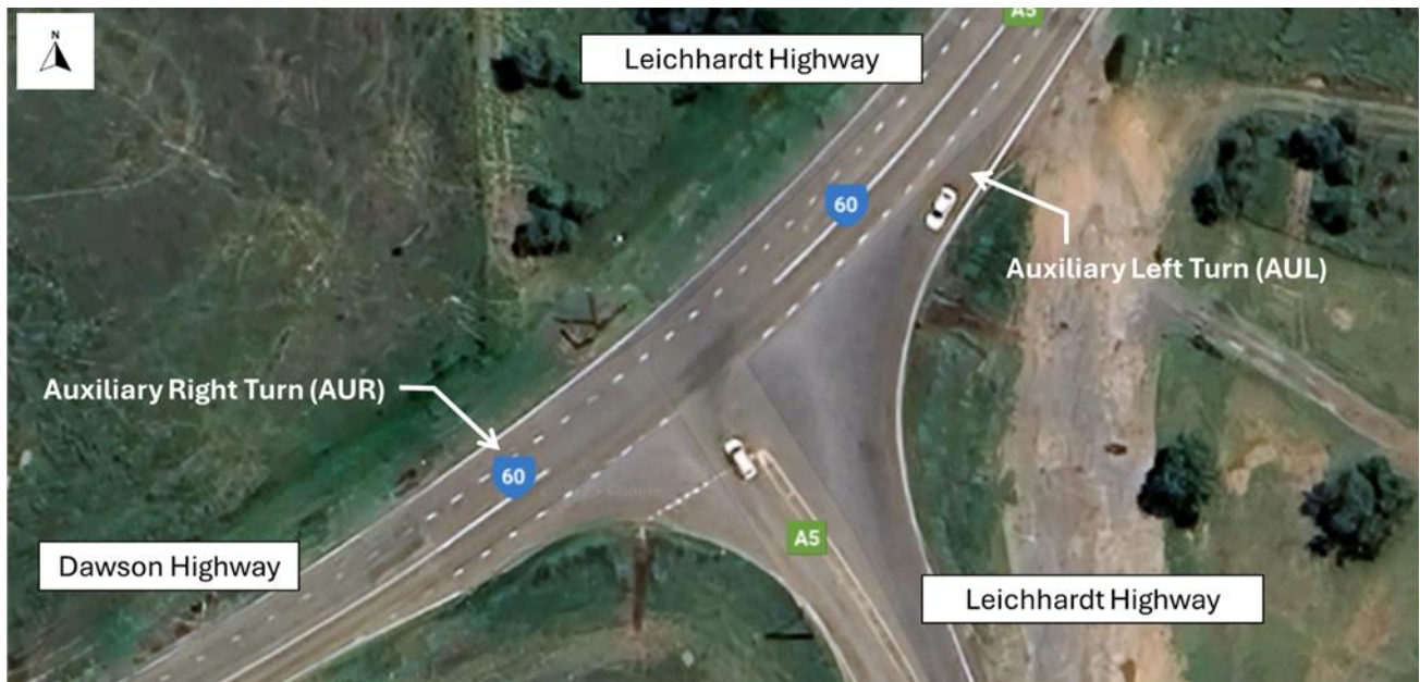
Figure 18.6 Leichhardt Highway/Dawson Highway intersection
