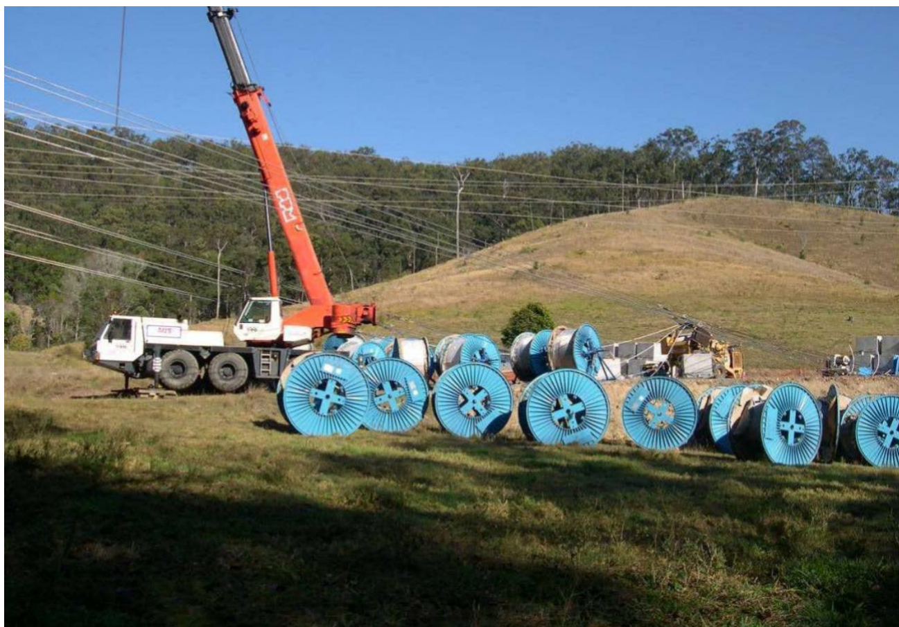
Figure 3.5 Transmission conductor drums and mobile crane utilised in structure erection
