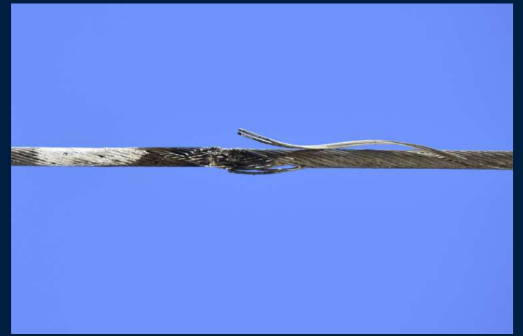
i Powerline critical infrastructure damage
